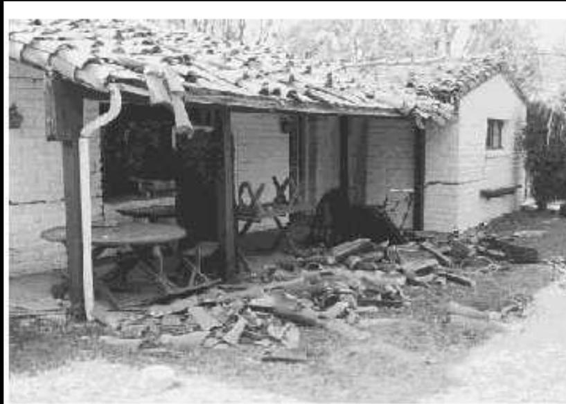
**Figure 10-11** A single-story residence that was subjected to very strong ground motions but suffered only moderate damage due to concrete bond beams and internal reinforcement.
